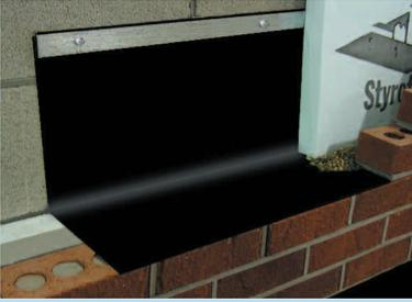
Use of off-the-shelf pressure bars expansion pinned onto CMU or screwed over metal stud sheathing.
