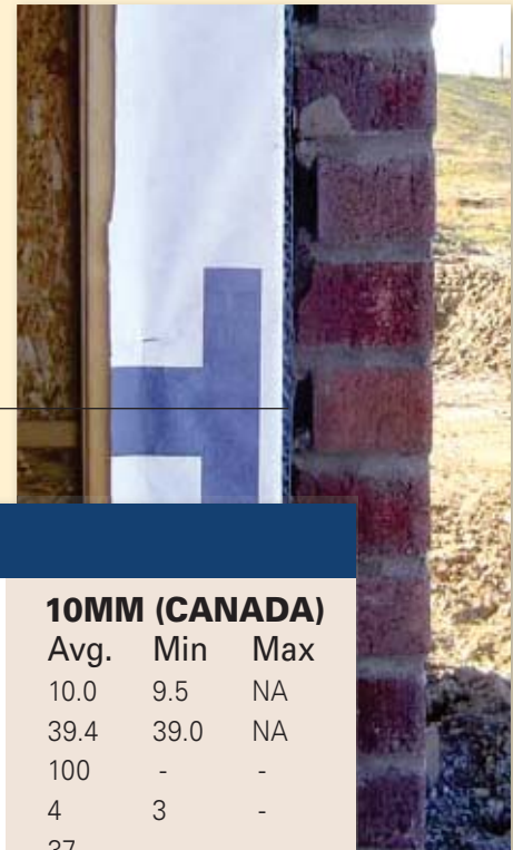
Figure #1 It is very important that a rainscreen come with a fabric adhered to the polypropylene to act as a mortar deflection. The absence of this fabric will cause the rainscreen to become clogged with mortar, making the polypropylene material almost useless.
