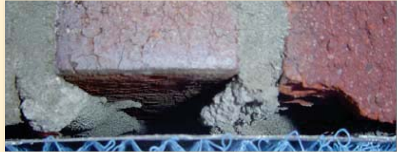
Figure #1 It is very important that a rainscreen come with a fabric adhered to the polypropylene to act as a mortar deflection. The absence of this fabric will cause the rainscreen to become clogged with mortar, making the polypropylene material almost useless.
