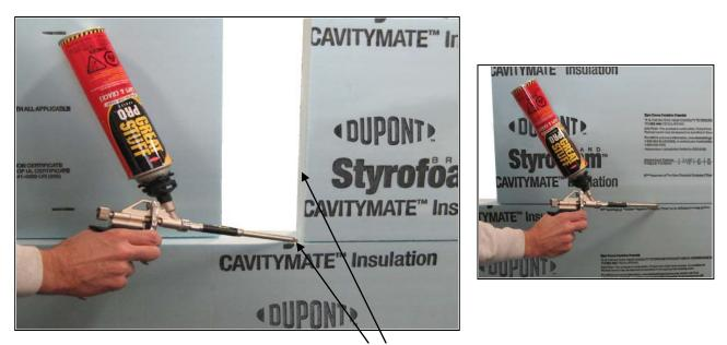
Place 1" diameter bead of Great Stuff Pro **adhesive/sealant** just inside the head and bed joint of the previously installed sheets.
