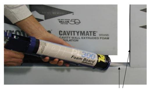
Place ¼" diameter bead of PL300 adhesive/sealant just inside the head and bed joint of the previously installed sheets.
