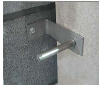
L Anchor w/Dowel - No Insulation
