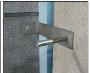
L Anchor w/Dowel with Insulation
