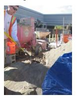
**NOTE:** In extreme cold conditions, a larger mass can be heated by creating an airspace between the top of the sand and the insulated blanket(s) by placing brick, CMU or rocks on top of the sand before covering it with insulated blanket(s) and a tarp.
